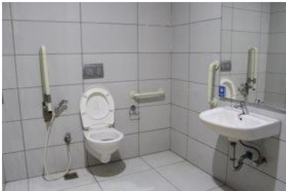
Picture 4: Installation of low-flow faucets, toilets
